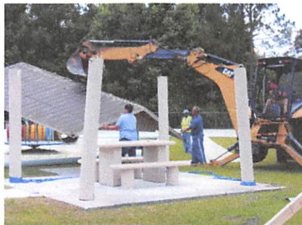
Public Works staff fixing a pavilion in the park
