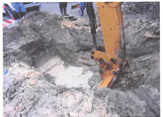
Delicate backhoe digging
