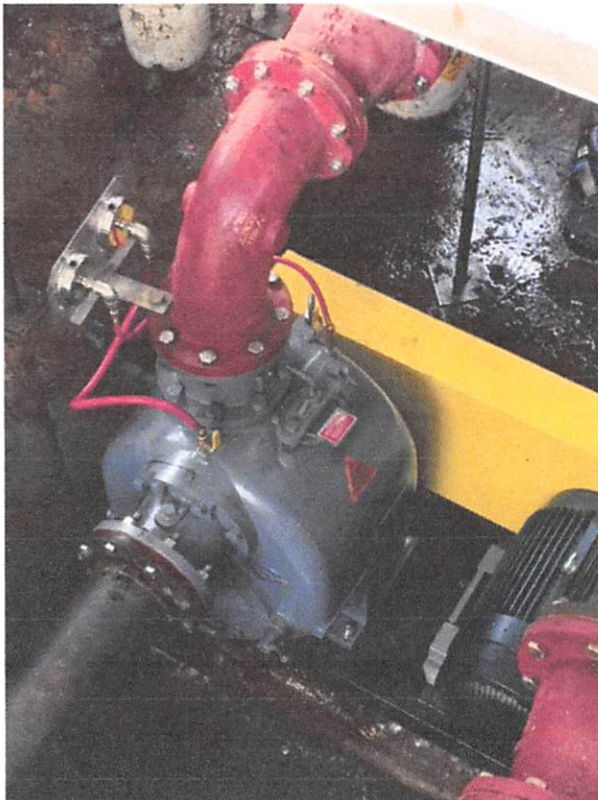
Lift Station Repair
