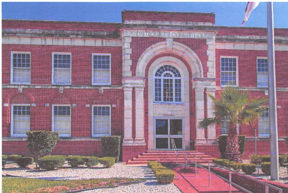
Union County Courthouse
