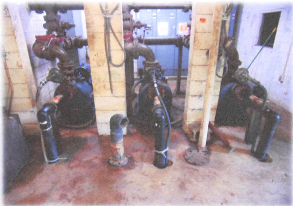
Wastewater main lift
